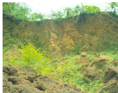
Fig. 2b. Tole landslide incidence in the western slopes of Mt Fako
