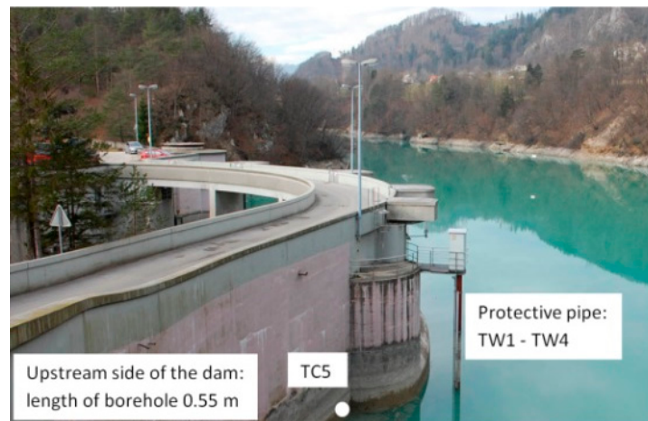
Figure 4. The locations of the temperature gauges on the upstream side of the dam and in the protective pipe (Photo: P. Žvanut).
