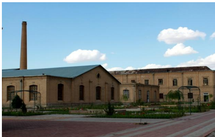
Fig. 3. The Building and Perimeter of the Khosravi Leather factory (authors, 2017)
