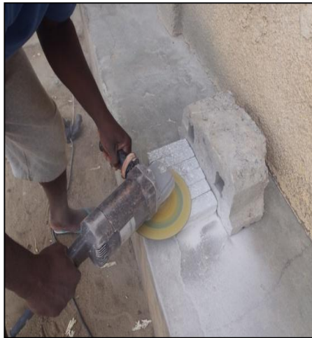
Fig. 3. Sanding operation
